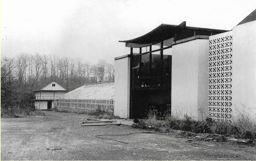
Loughran Gardens re-tail building with greenhouse and shed off to the left
