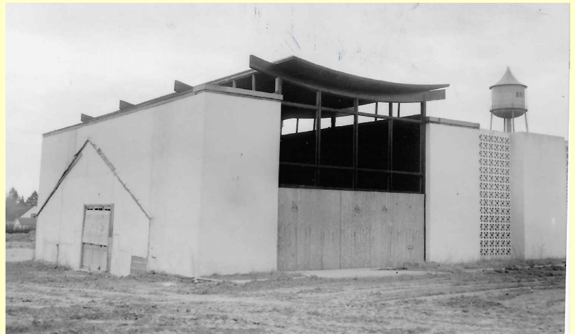
Retail building after the greenhouses were demolished (Note Brielle's old water tower in background)
